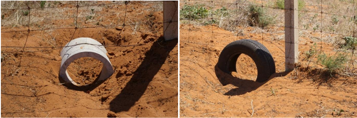
Figures 1 & 2: Examples of a concrete tunnel and car tyre utilised as wombat walkways
