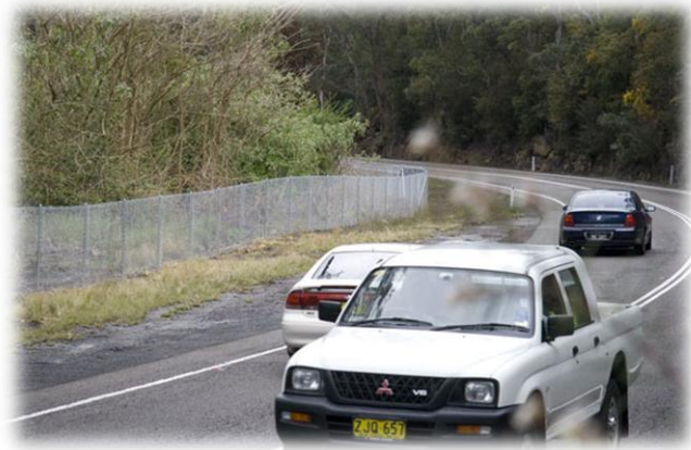
Figure 4 - The roadkill prevention fence on the Wakehurst Parkway 2007
