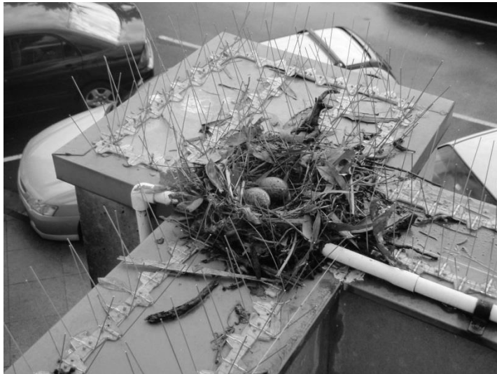
Seagull nest with eggs amongst bird deterrent spikes installed around rooftop edge – Frankston CAD 2011
