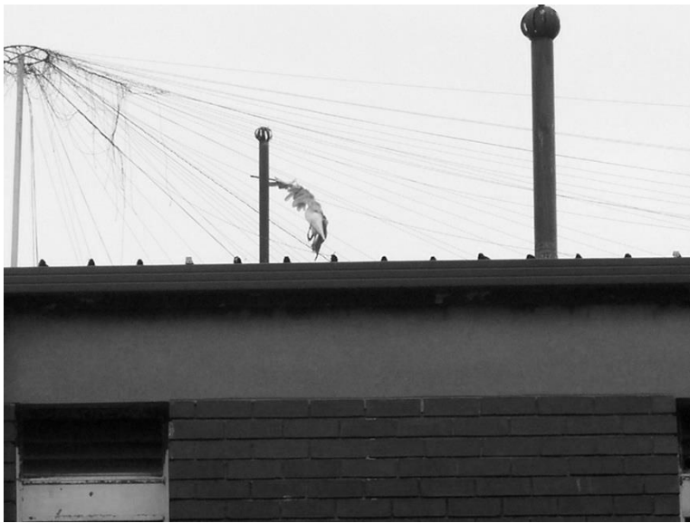
Dead gull entangled in loose crossing line deterrent system – Frankston CAD 2011
