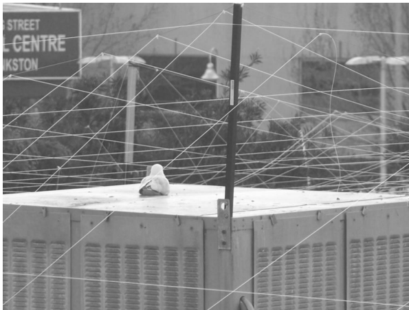
Gull sitting underneath an ineffective system – Frankston CAD 2012
