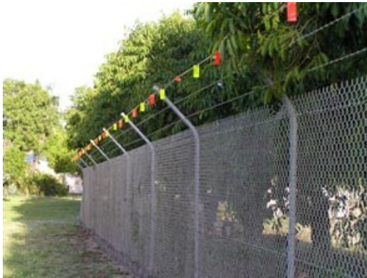
Photo: Jon Luly. Army Barracks Townsville.
